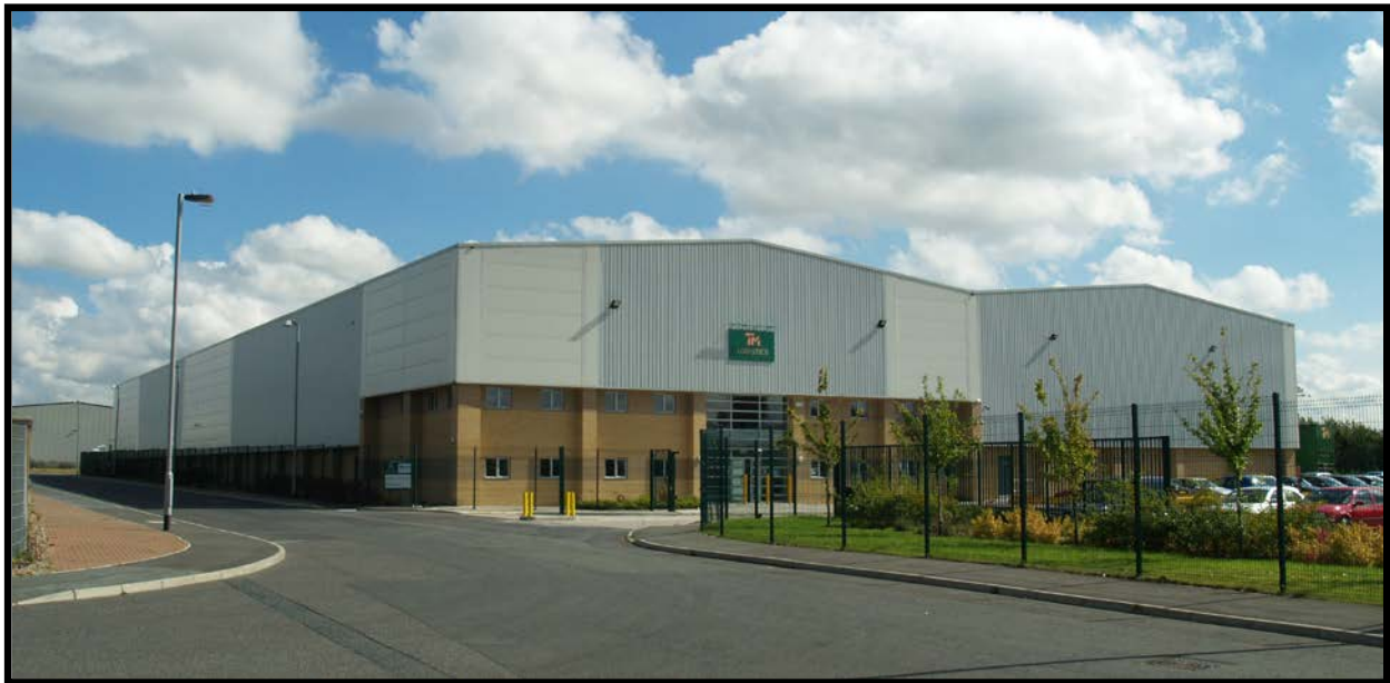
(Indicative Design – Photograph of Existing Phase 1 Unit)
